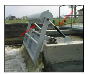
Stabilizing cylinders are oftentimes referred to as *steering stabilizers* in the automotive industry. Automotive steering stabilizers can be purchased at many local auto part stores such as NAPA or Sears and have been used by many irrigation districts on their ITRC Flap Gates.
