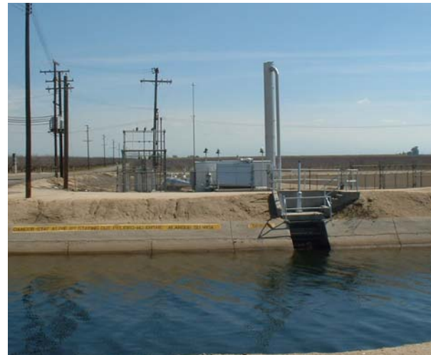
DEID turnout from the Friant Kern Canal that services an uphill section of the district.
