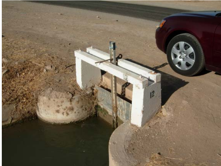
Figure 14. Imperial Irrigation District turnout. The gate opening and difference in head are measured for a known size of gate. The blue slip of paper in the hole near the top is left behind by the zanjero (operator) to let the farmer know the measurements and flow rate.
