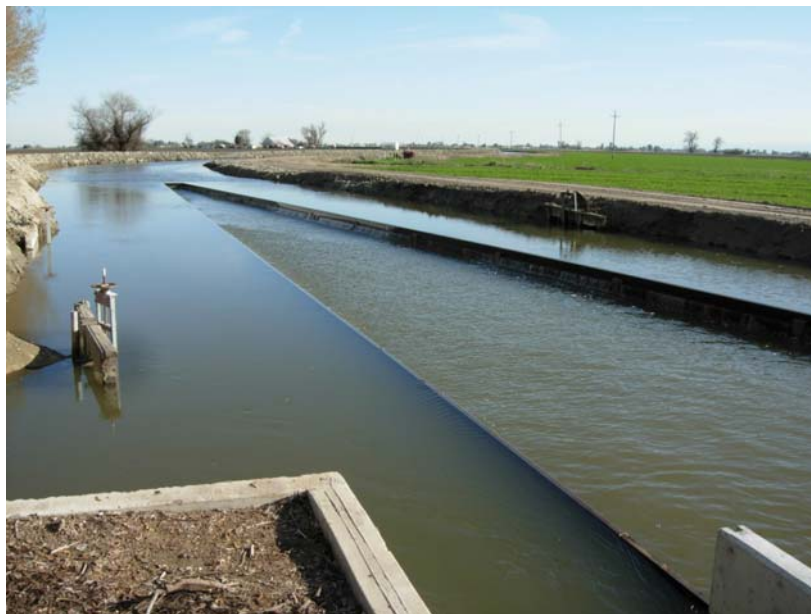
Figure 4. Very long, but simple, long crested weir at San Luis Canal Company. California has many hundreds of these structures.
