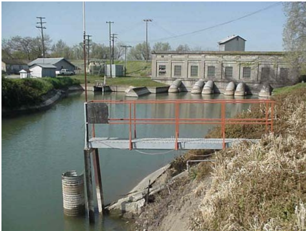
Figure 2. Tisdale Pumping Plant
