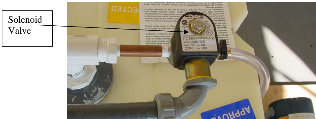
Figure 3: Normally closed solenoid valve
