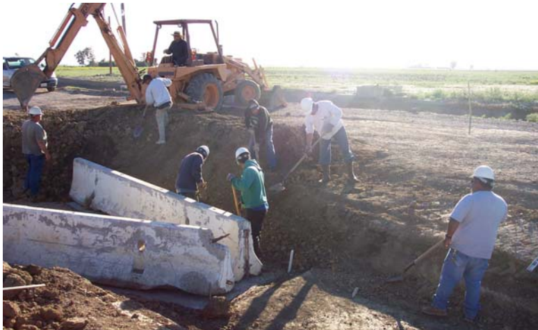
Figure 1. A long-crested weir being constructed with surplus K-rails (Banta-Carbona ID)
