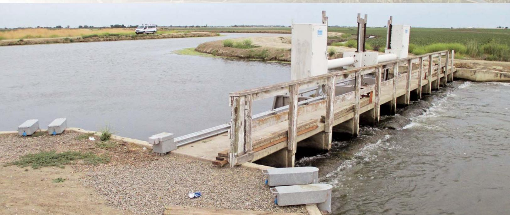
Modernization of an old canal check structure with new automated structures and special control logic
