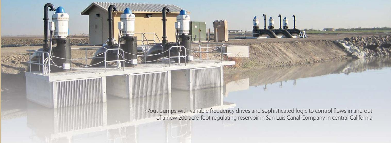
In/out pumps with variable frequency drives and sophisticated logic to control flows in and out of a new 200 acre-foot regulating reservoir in San Luis Canal Company in central California
