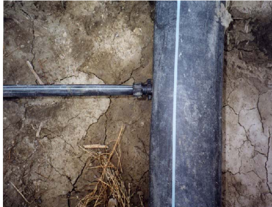
Figure 1. Manifold connection with "quick release" fitting directly connecting PE oval hose manifold to the tape.
