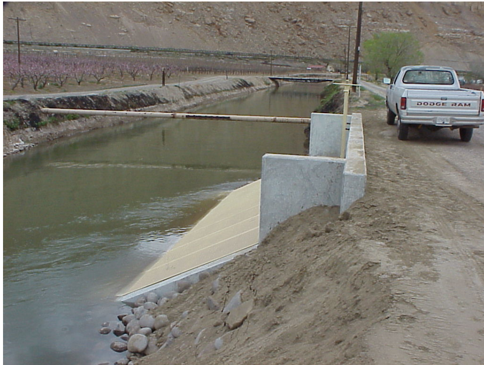
Figure 2. Palisade Pipeline Entrance
