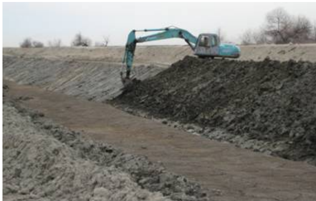
Figure 3. James ID Main Canal during side compaction
