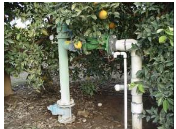
Figure 3. Automatic valve on a farmer turnout to shutoff deliveries before 12 pm and turn them back on after 6 pm.
