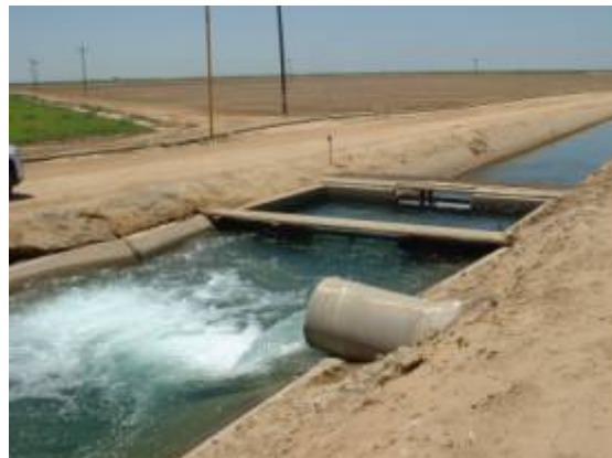
Figure 3. Water supply from a new reservoir supplying water to a canal during the on-peak period when the groundwater pumps are off.
