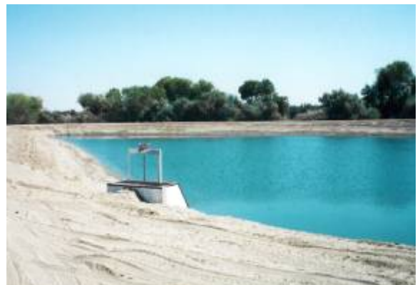
Figure 1. Gravity in – gravity out reservoir constructed to store water for use during the peak period
